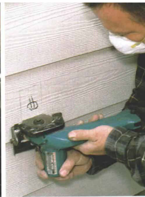
Plunge-cutting makes square holes.
